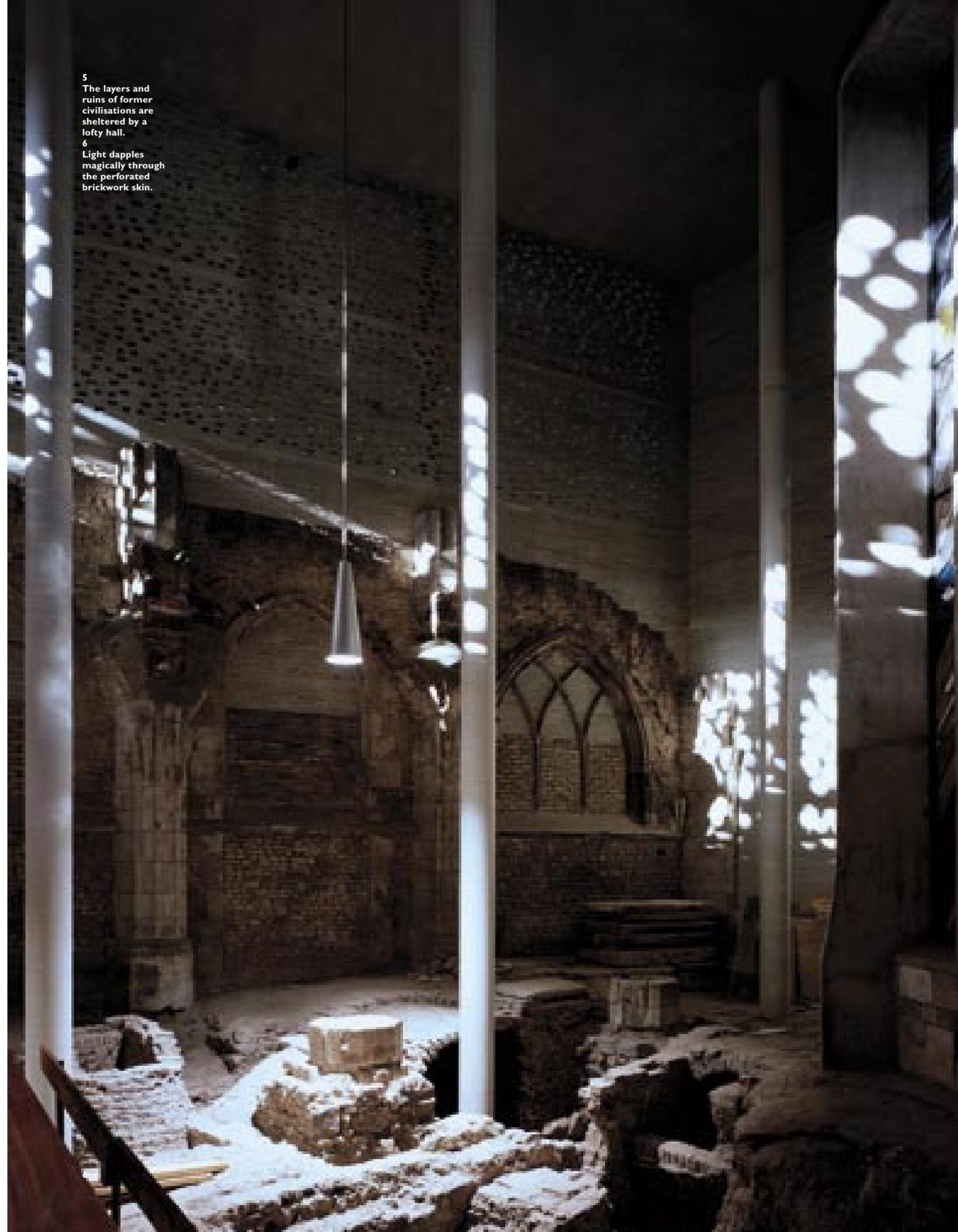
the building. The massive walls are partly made of hollow bricks to provide thermal insulation. To reduce thermal movement, they are kept at constant temperature by circulating water drawn from an aquifer 70m below ground, modified according to season. Air is drawn from the ruin hall heated or cooled and delivered to the galleries through their ceilings; exhaust is via a continuous slot round floor edges.
